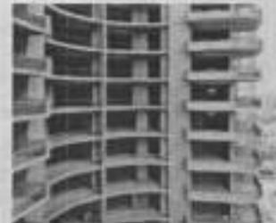
Tower A Raising Work
